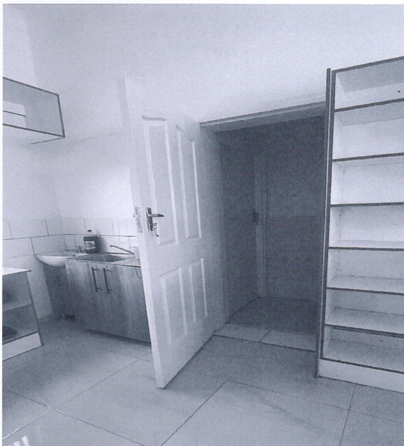
Picture 1 showing the newly installed door acting as a buffer between the toilet and dispensary area.
