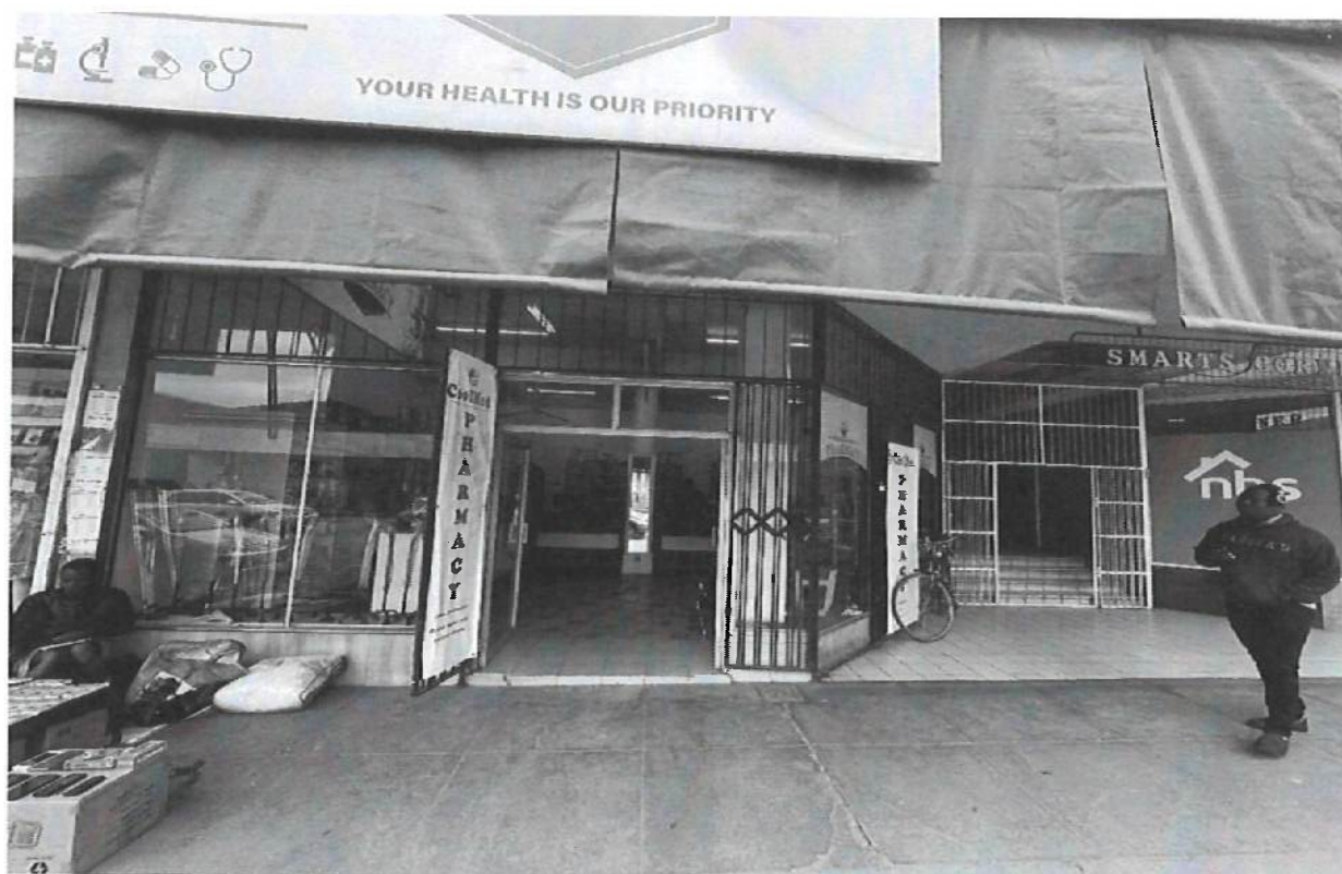
Image 2 depicting the glass windows without reinforcement from outside the pharmacy.
